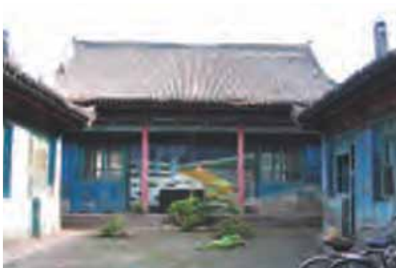
Top: Mijia Xiang Courtyard after GHF restoration; Middle: During restoration; Bottom: Before restoration. Photos: GHF
