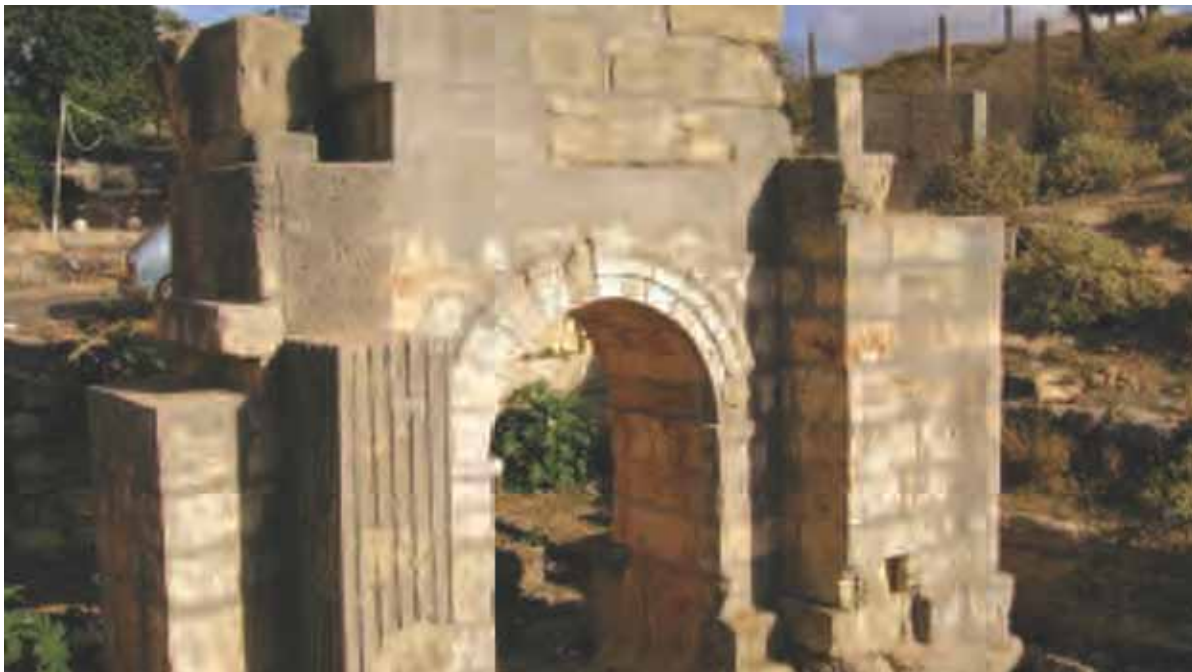
In Cyrene, Libya, a UNESCO World Heritage Site, Portland cement and rebar is used to patch together ancient monuments even today. Inappropriate reconstructions and unauthentic restorations for tourism are one of the most severe causes of loss and destruction to global heritage sites. Photo: GHF
