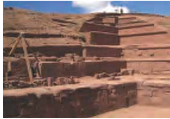
Insufficient Management: Bolivia's Akapana Pyramid may lose its UNESCO World Heritage status due to inappropriate restoration. Photo: Carla Windsor
