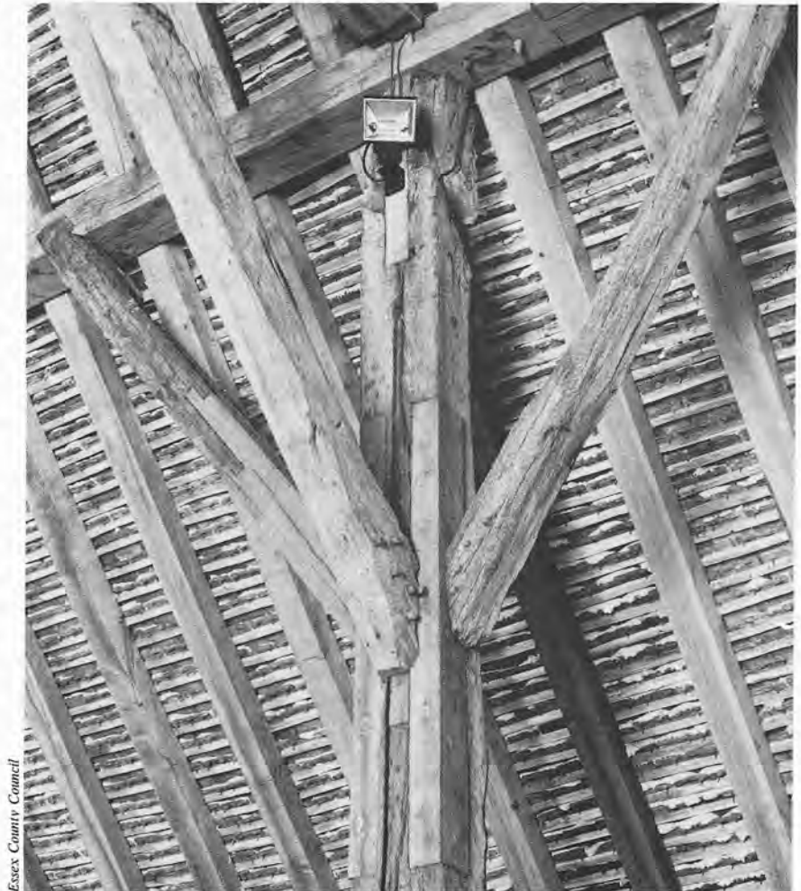
Myriad timber repairs to an early barn frame leaving much of the original timber remaining, and thus the evidence of structural changes in the past.
