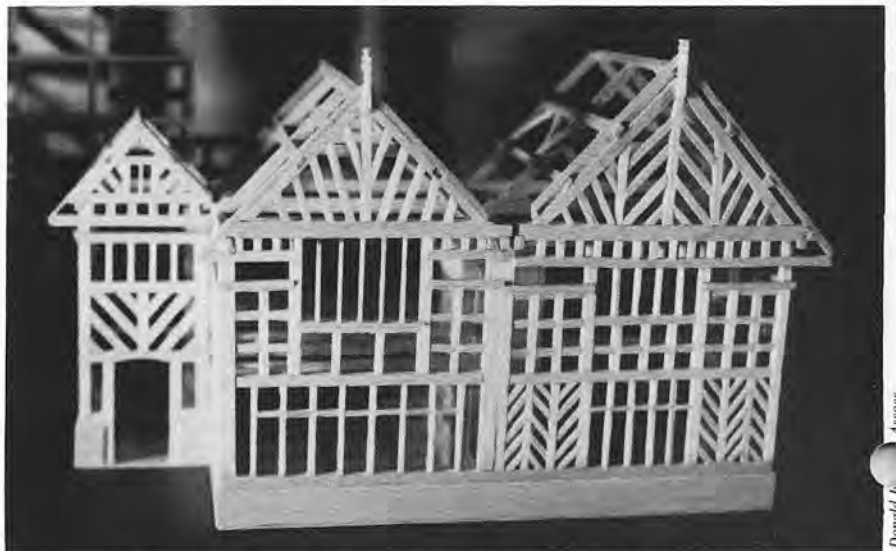
This model of timber-framing is a reconstruction of a building allowing the original construction and subsequent changes to be understood in context. The production of a model should be enough to satisfy any urge to 'restore' a timber frame to its original state; leave the building with its historical changes.
