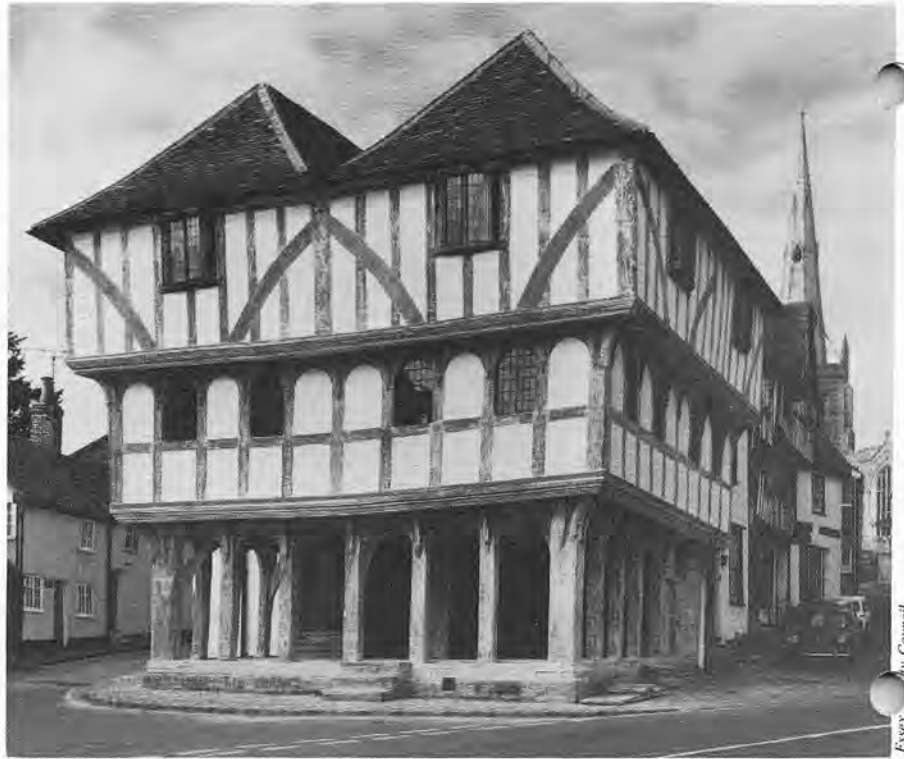
An example of conservative repair using traditional materials—all external wood and plaster surfaces were limewashed.
