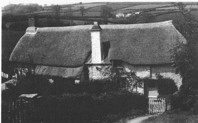
Fig. 6: The ridge peak is only found on a butt-up ridge; this is common in south west England
