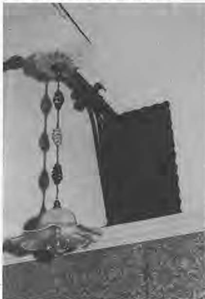
Fig. 18: Old luminaire at Standen: fittings like this must be retained in any rewiring. Note the correct use of a clear lamp.
