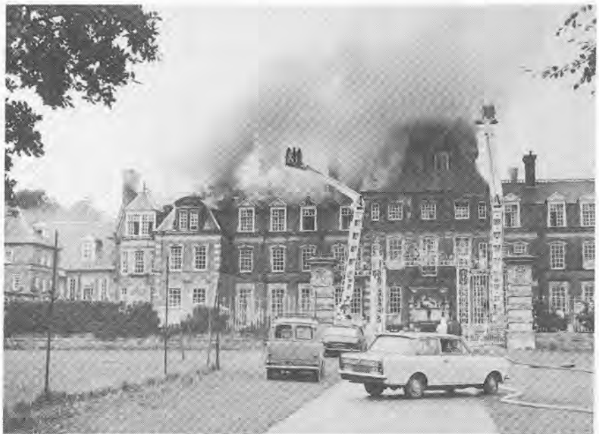
Clarendon School, Abergele, Clwyd: An example of the extensive spread of fire in a roof that was undivided internally
