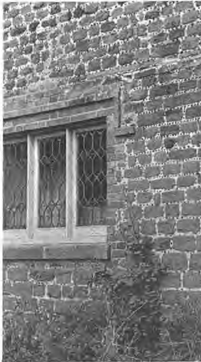
Carstone wall with galletting
