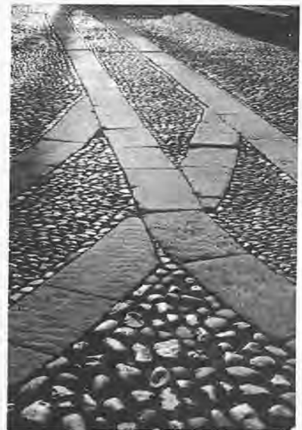
Paving, recently relaid in Queen's Gate, Chester (Donald Insall Associates)
