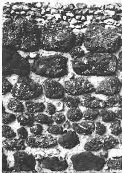
Two examples of walling, showing the possible variations in the thickness of mortar joints. Square knapped flint wall, Bridewell, Norwich. Rubble stone wall at North Elmham, Norfolk
