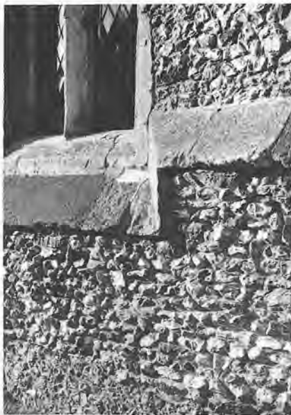
An example of flint walling with recessed pointing
