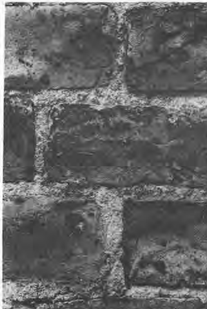
Original mortar still in good condition
