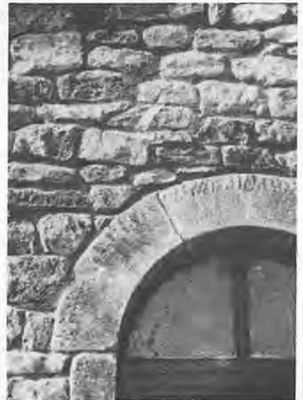
Slightly recessed pointing to emphasise the character of the individual stones
