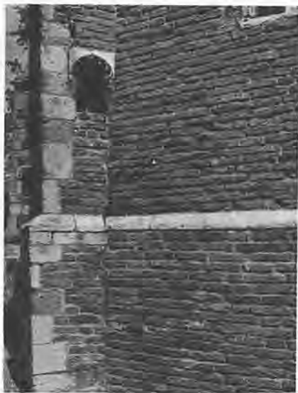
Recessed repointing below the string-course in character with original pointing above
