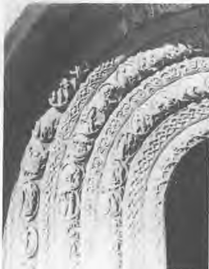
fig. 3: South Porch of Malmesbury Abbey. The cleaning here is a museum technique using pencil-sized air abrasive tools and very fine abrasives. The rate of working is essentially slow, and demands consistent patience and craftsmanship. Very vulnerable pieces of detail may need supporting with lime putty and stone dust, or fine lime grouting before later consolidation. Because the action of weathering and the aggressive activity of soluble salts continues, a subject of this value must remain under regular observation.
