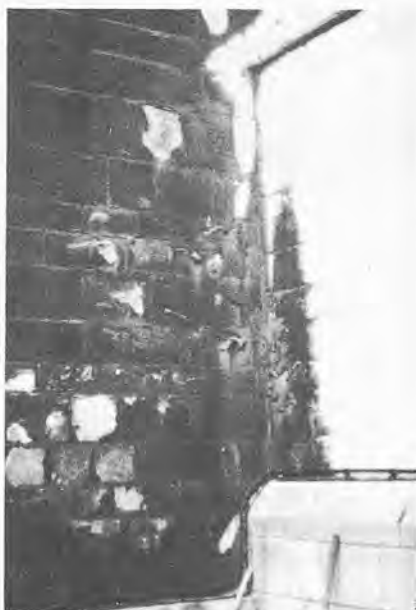
fig. 1: Soiling on old buildings is not something that can be ignored. A decision must be made on whether or not the dirt deposits are harmful and whether they should be wholly or partly removed. If they are to be removed, what is the correct method and are the skill resources available adequate to carry out the work sensitively and safely? A building of the complexity of Henry VII's Chapel at Westminster cannot even be examined properly without the removal of some of the dirt, which builds up into encrustations of a positively harmful kind. The detail (left), from the Palace of Westminster, shows splitting and spalling sulphate skins on sheltered limestone contrasting with the sound, regularly rain-washed surface adjacent. Natural weathering effects in a polluted environment often present a strong case for maintenance washing.
