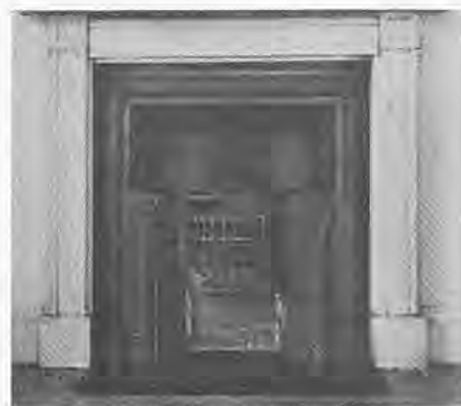
Above: A typical hob grate at 94 The Mount, York, North Yorkshire, the fireplace is on the first floor
