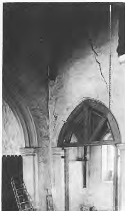
fig 19: The effect of the drawing away of the tower on one of the nave arches at Puttenham church, Hertfordshire
