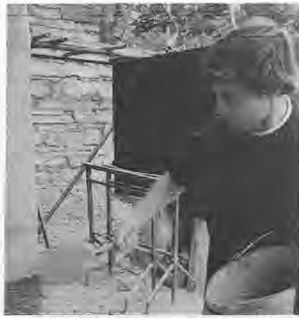
Rough-cast being applied with a wristy backhand flicking motion.
