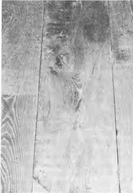
Warmth and richness of a well-repaired old floor.
