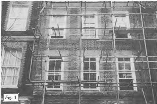
An area of completed tuck-pointing. 7-9 Great Ormond Street.
