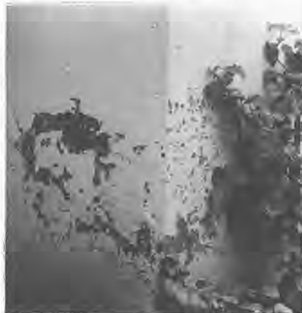
A modern paint coating, consisting of fine aggregate bound with resin, spalling less than two years after application to an 18th century wall.
