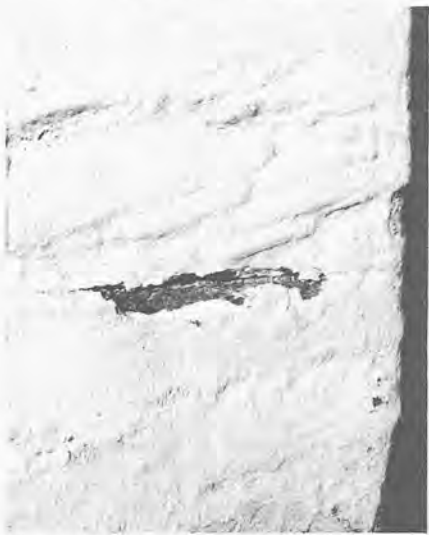
Moisture trapped behind an impervious paint film has caused it to blister. The effect of salts and frost has led to further decay.
