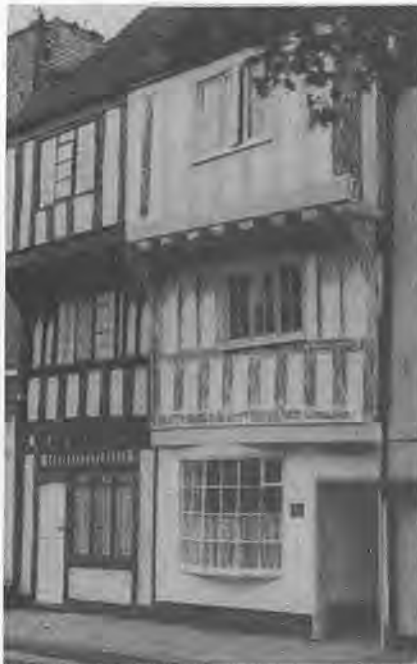
The Society advises against blackening timbers in favour of limewashing both timber and panel. Numbers 82 and 83 Church Street, Tewkesbury, demonstrate the subtlety of the latter.
