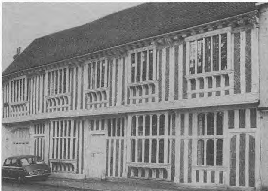
At Paycocke's in Coggeshall, Essex, the timbers were limewashed leaving the brick nogging exposed. This photograph was taken when the work was first carried out. The effect is startling. After three years, however, the oak weathered to a superb-looking silvery colour.
