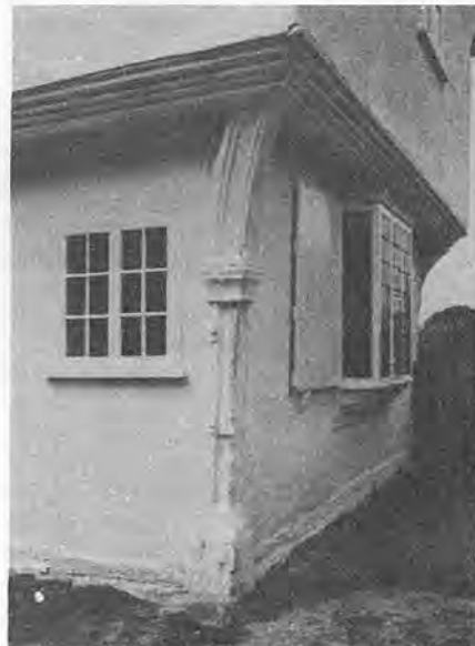
At Paycocke's in Coggeshall, Essex, the timbers were limewashed leaving the brick nogging exposed. This photograph was taken when the work was first carried out. The effect is startling. After three years, however, the oak weathered to a superb-looking silvery colour.
