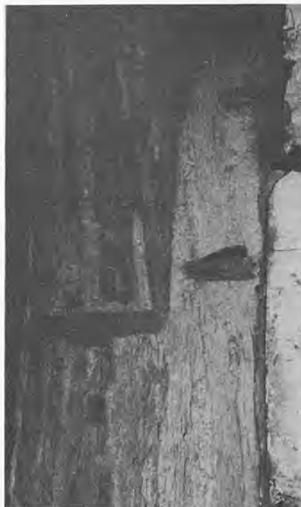
The result of defrassing a main post which was originally covered with C16 painted decoration. This decoration once formed part of a scheme covering all wall surfaces—plaster and timber.
