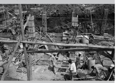
Figure 11: Multi-storey buildings in Addis Ababa are typically constructed from cast in-situ reinforced concrete frame with brick infill walls. © UN-HABITAT
