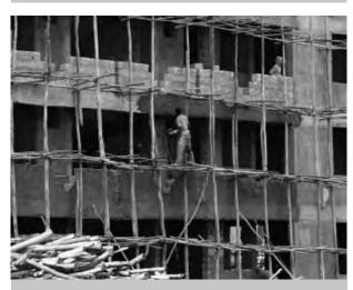
Figure 28: Workman applying plaster to the first-storey of a condominium block. Bole Summit, Addis Ababa.
