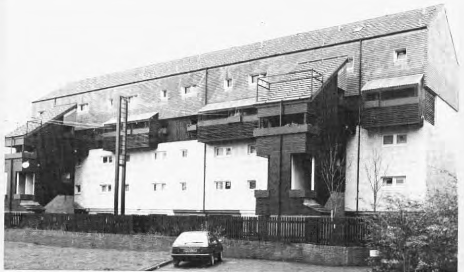
Changes made to original structures showing: Top: new entrances provided to lower maisonettes; Centre: new south facing balconies; Bottom: new staircases, clothes drying facilities and external cladding.
