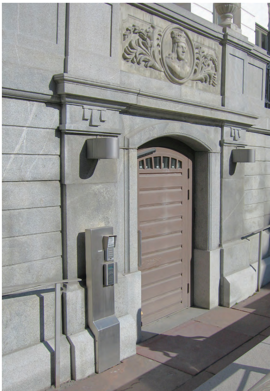
FIG 8-5. The new adjusted entrance is equipped with a new outward going door with automatic opening door opener, handrail, armatures and a post for entry control. O. Isola ©
