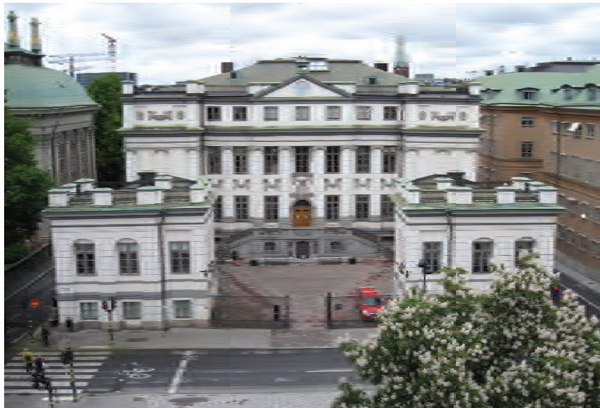
FIG 8–1. Bondeska palatset, southern façade after the interventions in 2004. The courtyard surface consists of cobblestones with paths of sandstone and markings with setts. Oiva Isola ©
