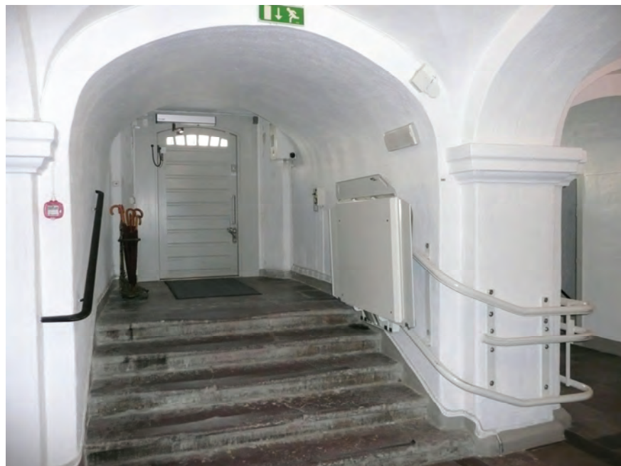
FIG 8–7. The new door to the personnel entrance is fitted with an automatic door opener. The stair lift is in an uplifted position. Oiva Isola ©
