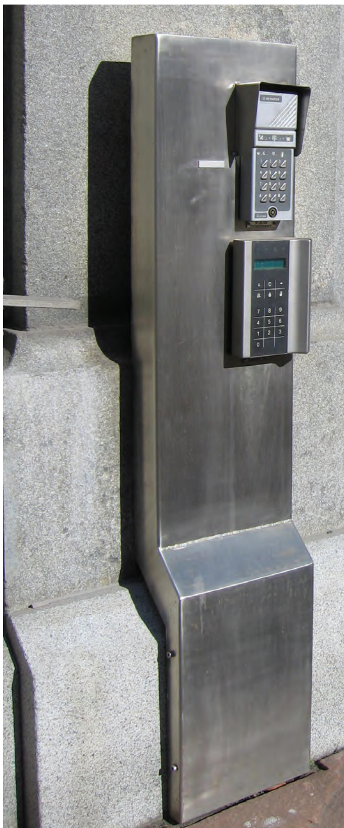
FIG 8–6. The post with elbow switch, buttons for entry code and entryphone have been installed at a distance from the wall and attached only to the ground. O. Isola ©
