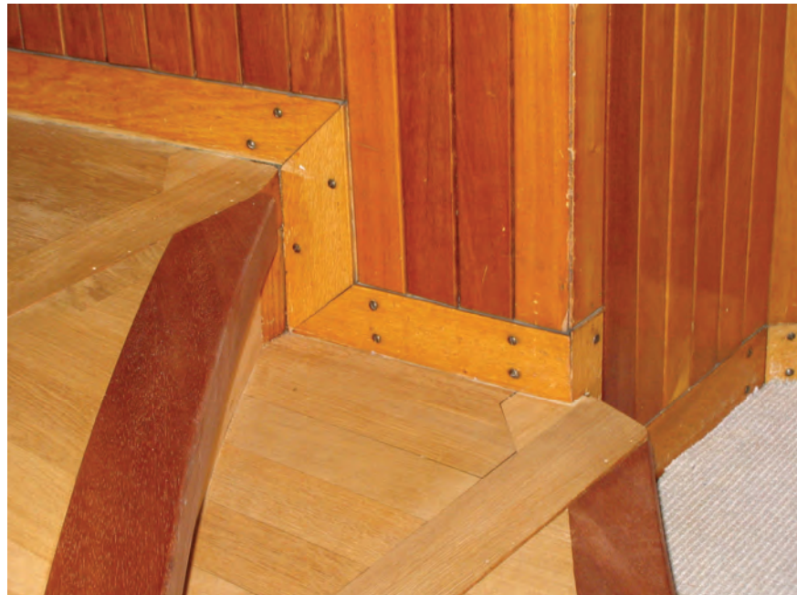
FIG 13-5 Detail showing how the new ramp meets the existing step. Alice Rosenberg ©
