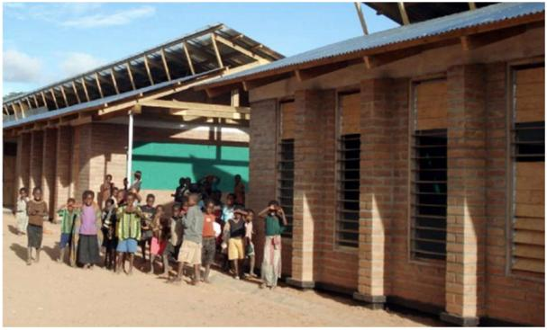
Key data compressed stabilised soil blocks, Cinva–ram block press, site-won soil 290mm×140mm×100mm load-bearing single-storey reinforced concrete floor slab with fired brick foundation Damp-proof course and termite nib.
