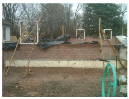
Figure 10. Window Bucks Installed
