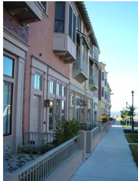
Figure 33: Live-work homes, Hercules, California
