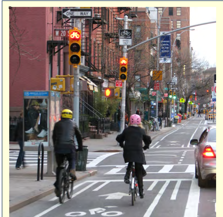
Exhibit 4-14: 9 th Avenue bicycle lane in New York City. A dedicated bike lane with separate traffic signals separates bicyclists from vehicles on city streets.
