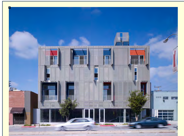
Exhibit 4-17: Cherokee Mixed-Use Lofts in Hollywood, California. This residential and retail building is 40 percent more efficient than required by California's building code; has a green roof, water-efficient fixtures, drought-tolerant landscaping, and solar heating; and uses materials throughout that are recycled and contain low or no VOCs. It is close to shops, services, and other amenities so residents can walk for many daily needs. Photo source: Calderoliver via Wikipedia Commons
