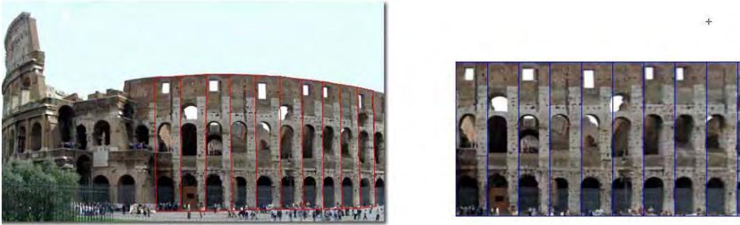
*The curved surface of the Colosseum has been transferred to a plan using a mesh of points which are shown in red on the original photo and in blue on the final result.*
