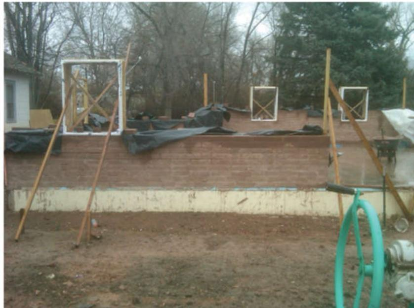
After the door bucks are set, the first course of CMU blocks or CEBs, based on the design for the area climate, can be laid directly on the foundation. For CMUs, this step is usually done with cement or mortar. For CEBs, a contractor grade construction adhesive affords the best bond
