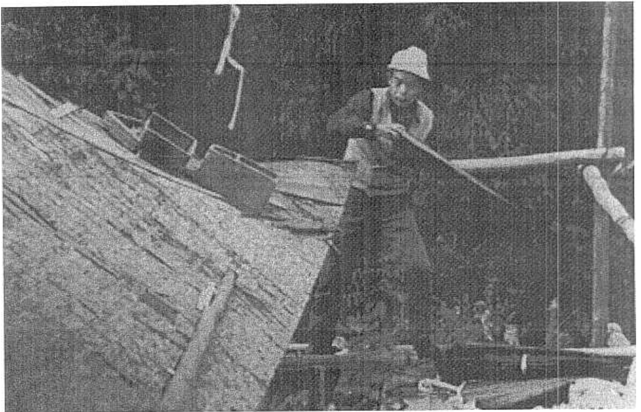
Illustration 4: Traditional roof repair in the temple of Cyōjūji in Japan. Traditional skills are recognized in Japan as part of the national cultural heritage, and their continuation and survival are given special attention.
