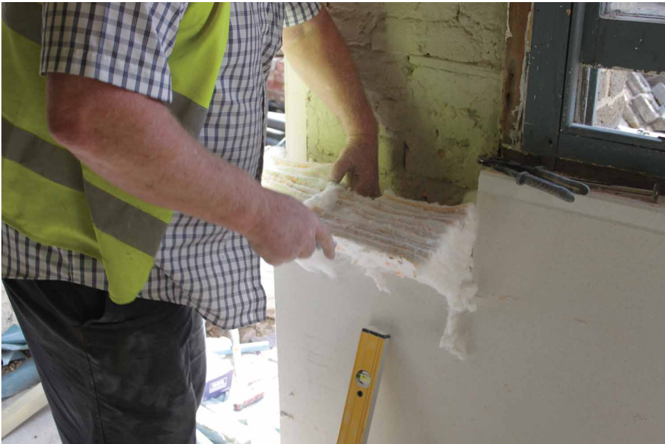
Figure 12. Aerogel insulation. (Credit: National Trust Picture Library/Jon Whitehead).
