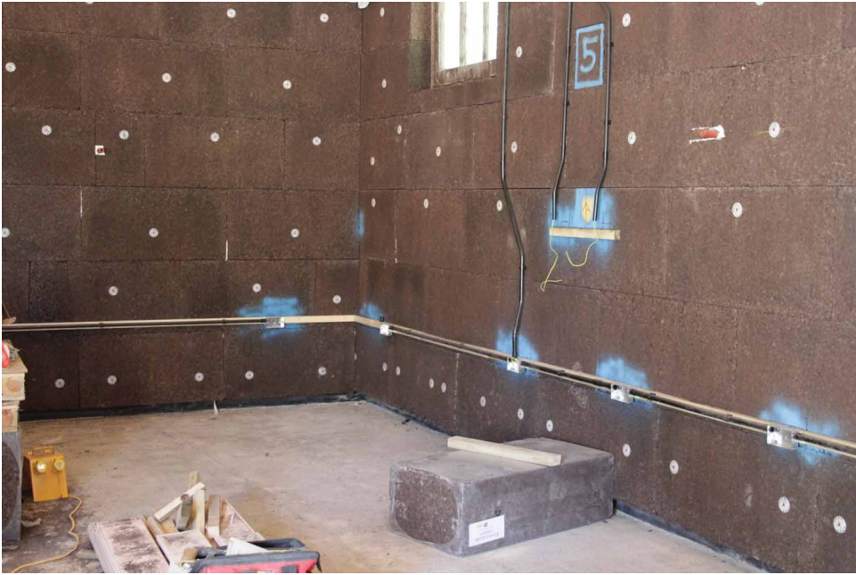
Figure 11. Cork insulation. (Credit: National Trust Picture Library/Jon Whitehead).
