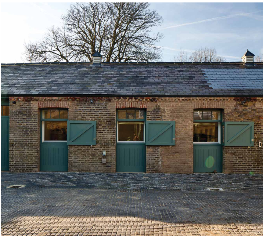
Figure 8. PV slates. (Credit: National Trust Picture Library/Jon Whitehead).
