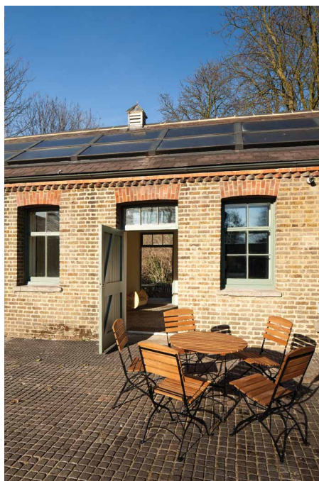
Figure 9. PV-T panels, café tables and original windows. (Credit: Louis Sinclair).
