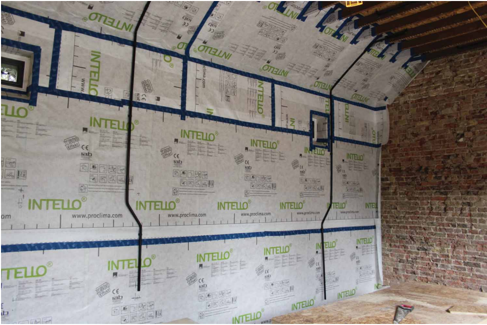
Figure 13. Intelligent membrane. (Credit: National Trust Picture Library/Jon Whitehead).
