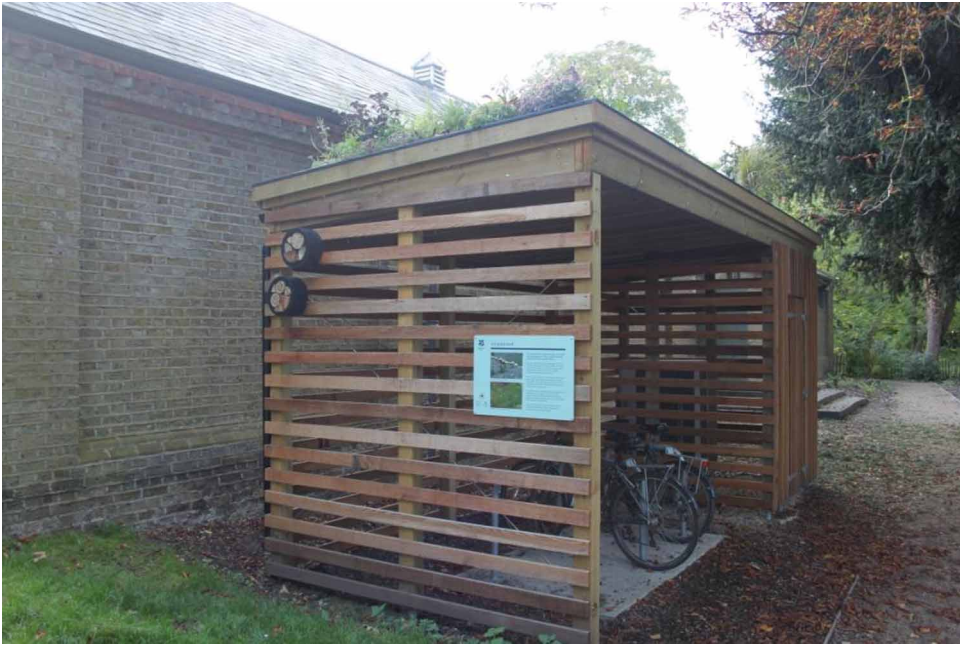
Figure 10. Air source heat pump in cycle shed with living green roof. (Credit: National Trust Picture Library/Caroline Pankhurst).
