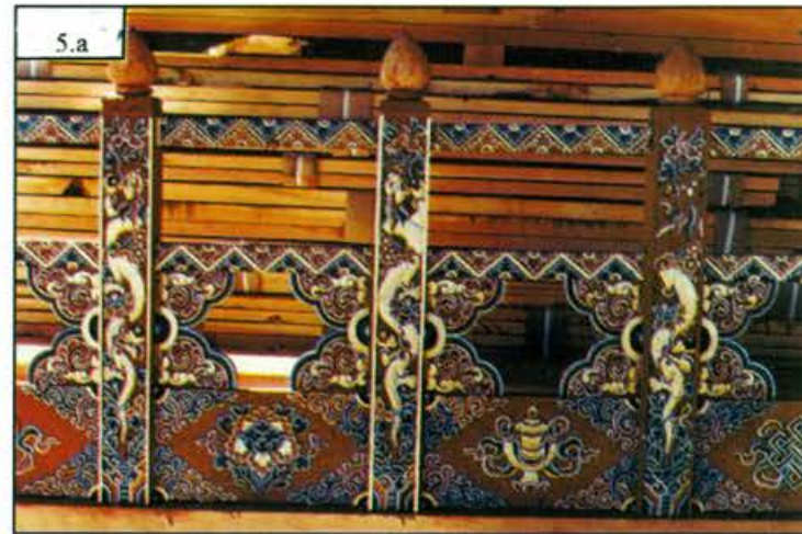
Photo 5.a shows the Tazi with Tshegay and Photo 5.b without Tshegay . Both are permitted.
