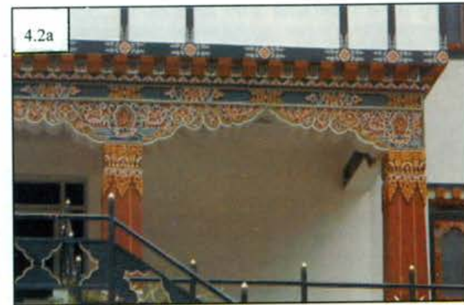
Photo 4.2a - The tail of the crossing Zhu , Dhung and Pedma at the corner is missing. It should look like in photo 4.2b.
