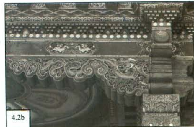
Photo 4.2a - The tail of the crossing Zhu , Dhung and Pedma at the corner is missing. It should look like in photo 4.2b.
