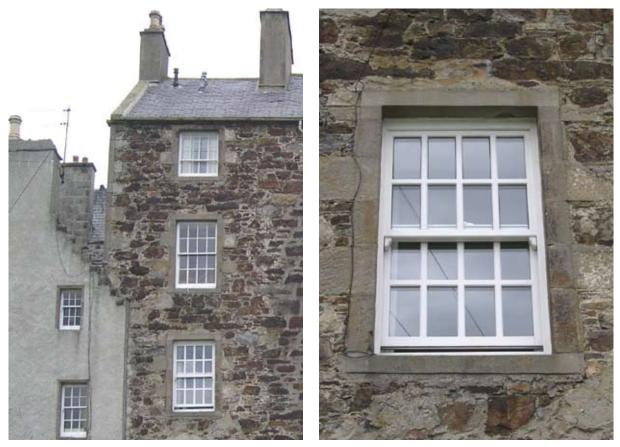
Illus 3.15(a), (b) Replacement PVCu double glazed sash and case window (bottom window in exposed rubble wall). While resembling the timber sash and case window above, the wider frame and glazing bars detract from the character of this Category B listed building (1790) converted into apartments. (Photo: D Urquhart).
