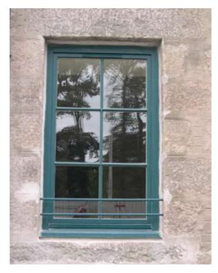
Illus 3.16.1 New window frame fixed into resized opening in this former mill converted to apartments. Note the rather poorly executed mortar pointing around the repositioned stone cill.
