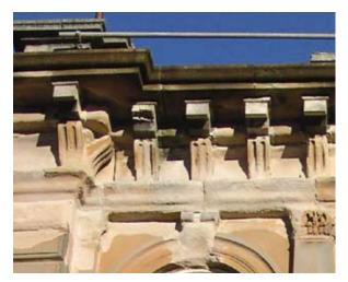
Illus 2.3. An example of inappropriate replacement elements is illustrated on this B listed building. Stone brackets supporting the stone cornice have been replaced with reinforced precast concrete brackets. The reinforcement is corroding creating a risk of falling masonry. An original stone balustrade supported on the cornice has been removed. (Photo: D Urguhart).
