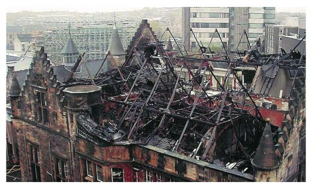
Illus 2.4.1 The presence of large, uncompartmented roof voids has resulted in severe fire damage to the roof and interior of this Category A listed university building. (Picture by Leigh Johnston, Historic Scotland and reproduced here from TAN 28).
