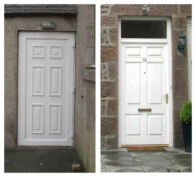
Illus 3.16(a) The door on the left is an inappropriate modern replacement plastic door in this traditional 1914 building (Photo: D Urquhart).
