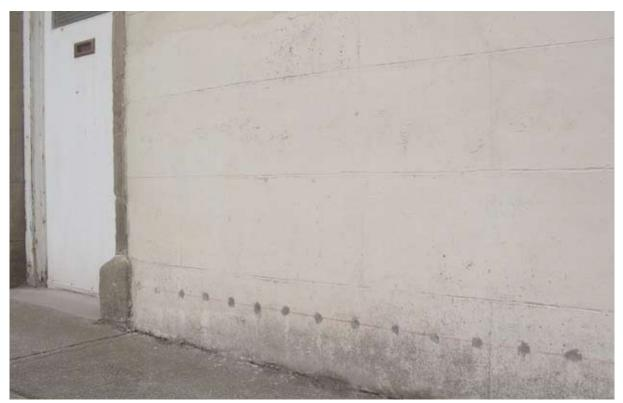
Illus 3.4.2 Damproofing inserted into a historic wall, circa mid-C19 (listed Category C(S)) (Photo: D Urquhart). Note: In this example it is likely that the dampness problem has been exacerbated by the application of hard cement render and the installation of a new concrete ground floor on a DPM. The rear wall of the building is unrendered rubble, which has not had a DPC installed.
